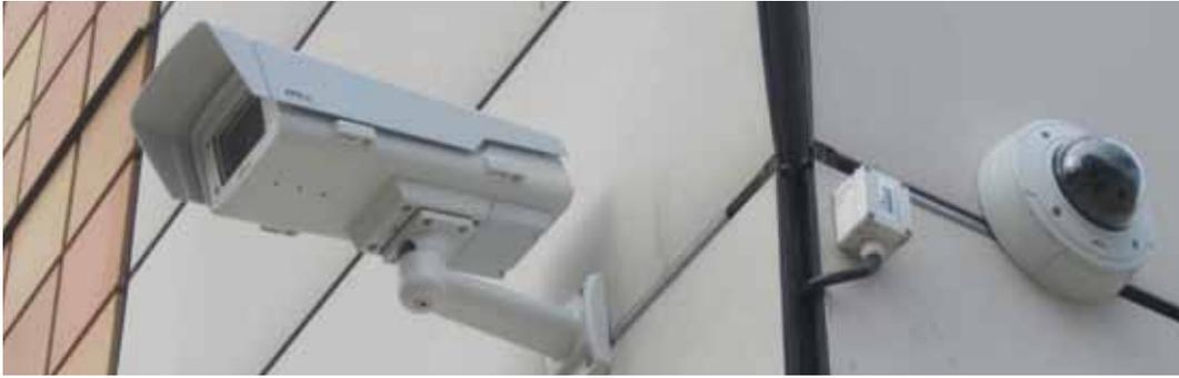
The solution at Gersager Park consists of AXIS Q1755 and AXIS M3204 Network Cameras that monitor public pathways and tunnels that lead into the housing area.
