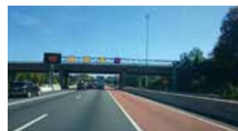
Shoulder closed to traffic (red cross dynamic sign)
