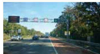
Shoulder open to traffic (green arrow dynamic sign)
